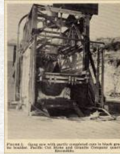
Figure 3. Gang saw with partly completed cuts in black granite boulder. Pacific Cut Stone and Granite Company quarry, Escondido.
